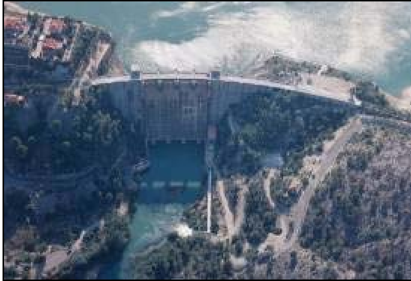
Figure 1. The study dam and reservoir.
