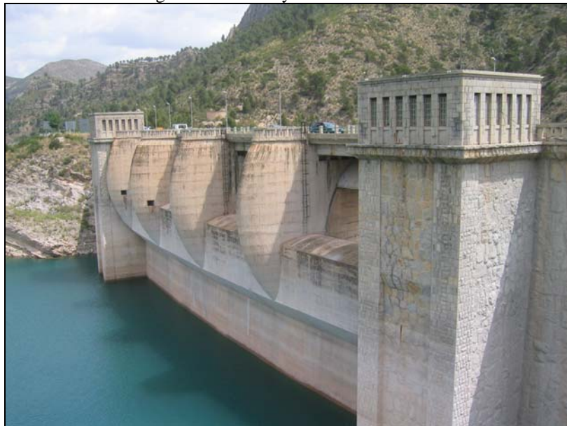
Figure 2. The main spillway from upstream.
